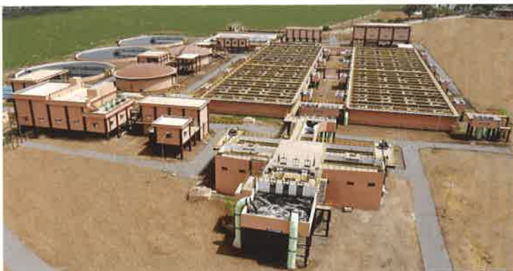
84 MLD Two Stage Biological (UASB + MBBR) STP at Variav for Surat Municipal Corporation
