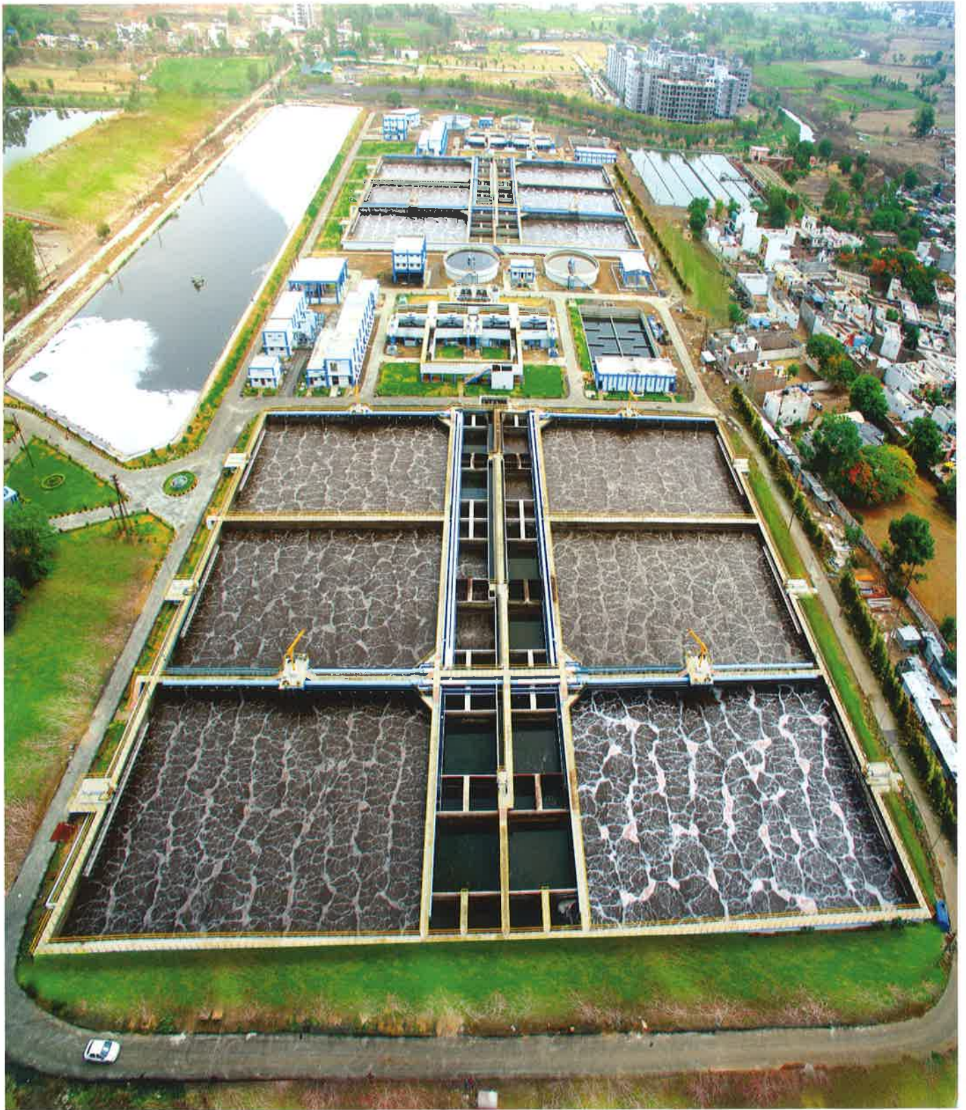
245 MLD STP for Indore Municipal Corporation, World's first Largest Single Stage Biological SBR Based STP
