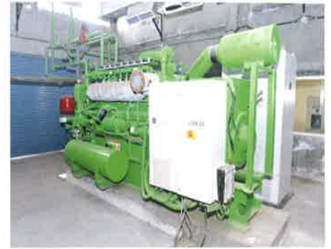
600 KWe Capacity Bio Gas Power Plant at 84 MLD STP, Variav for SMC, Surat
