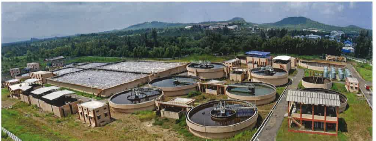
15 MLD CETP for Gujarat Industrial Development Corporation, Sarigam , Vapi
