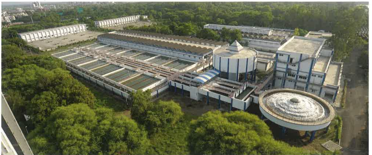
200 MLD WTP at Sarthana for Surat Municipal Corporation
